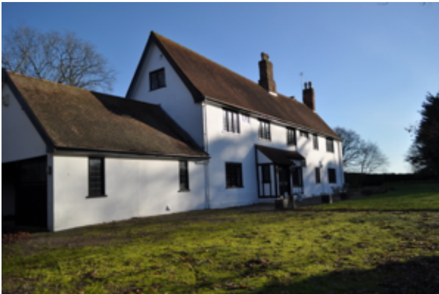
Farnham Manor, owns Ancient Woodland/CWS Pond Wood and a Walled Garden; 10m and 20m distance from EDF's site boundary and completely exposed.
